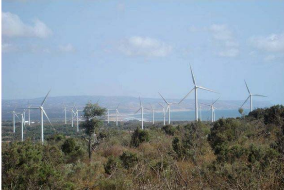
Picture 5: Non geometrical location of wind turbines may be a good choice in wild areas such this case in Morocco
